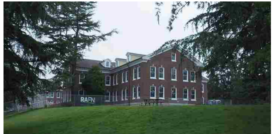
Figure 42. The Mercy affordable housing, located in the west of Building 18
