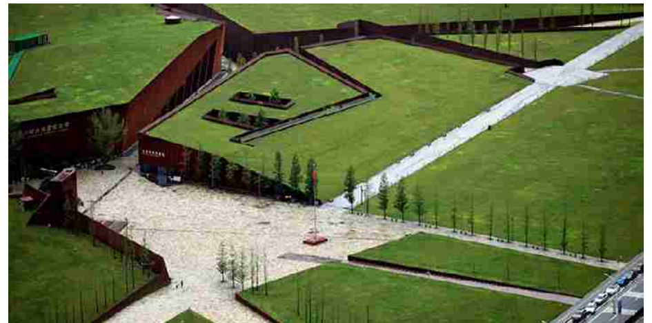
Figure 18. Wenchuan Earthquake Memorial Museum in Anren, Sichuan, China | Cai Yongjie. Source: Designboom
