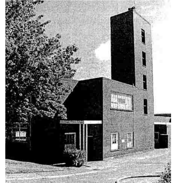
Figure 32. South side of the building. Source :Sand Point Magnuson Park Building 18 Firehouse Studio Project Feasibility Study Report By Arc Architects, page 10
